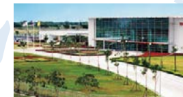
Toyota Motor Asia Pacific Engineering and Manufacturing Co., Ltd. Thailand (Samut Prakan Province)
