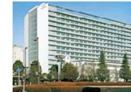
Head Office Technical Center Japan (Toyota City, Aichi Prefecture)
