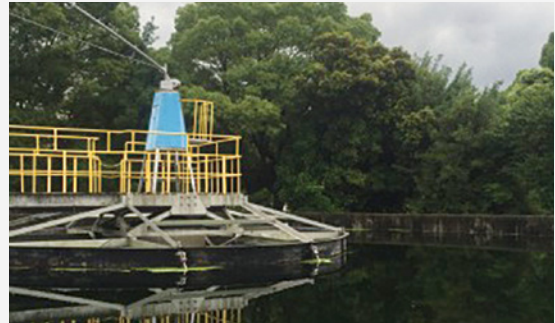
Wastewater treatment facility
